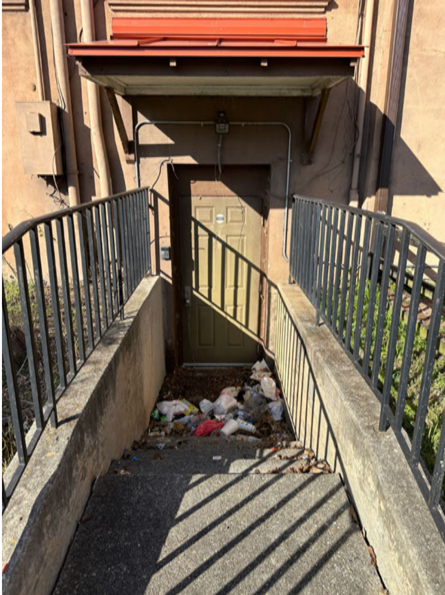
PHOTO: 5 S8 — South Elevation
