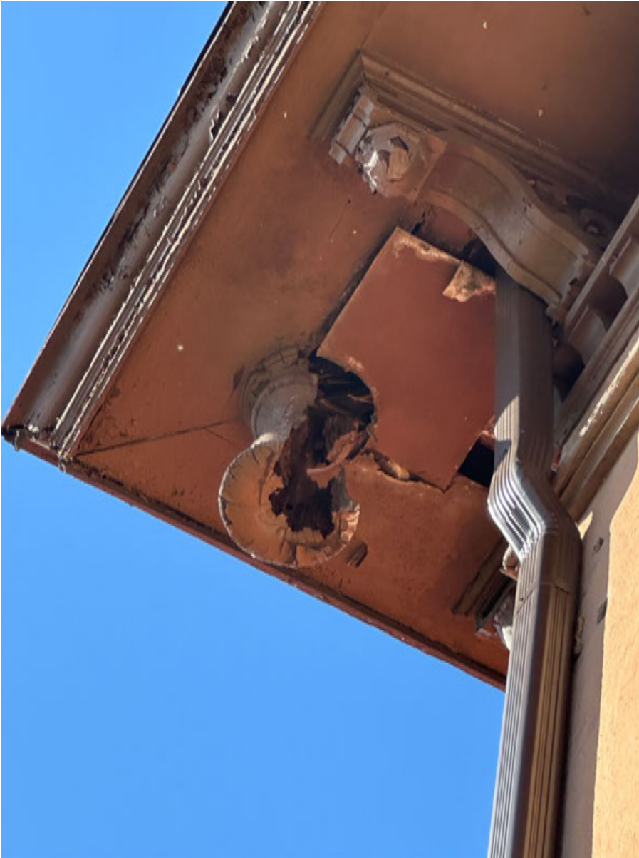
PHOTO: 8 E2 — East Elevation
