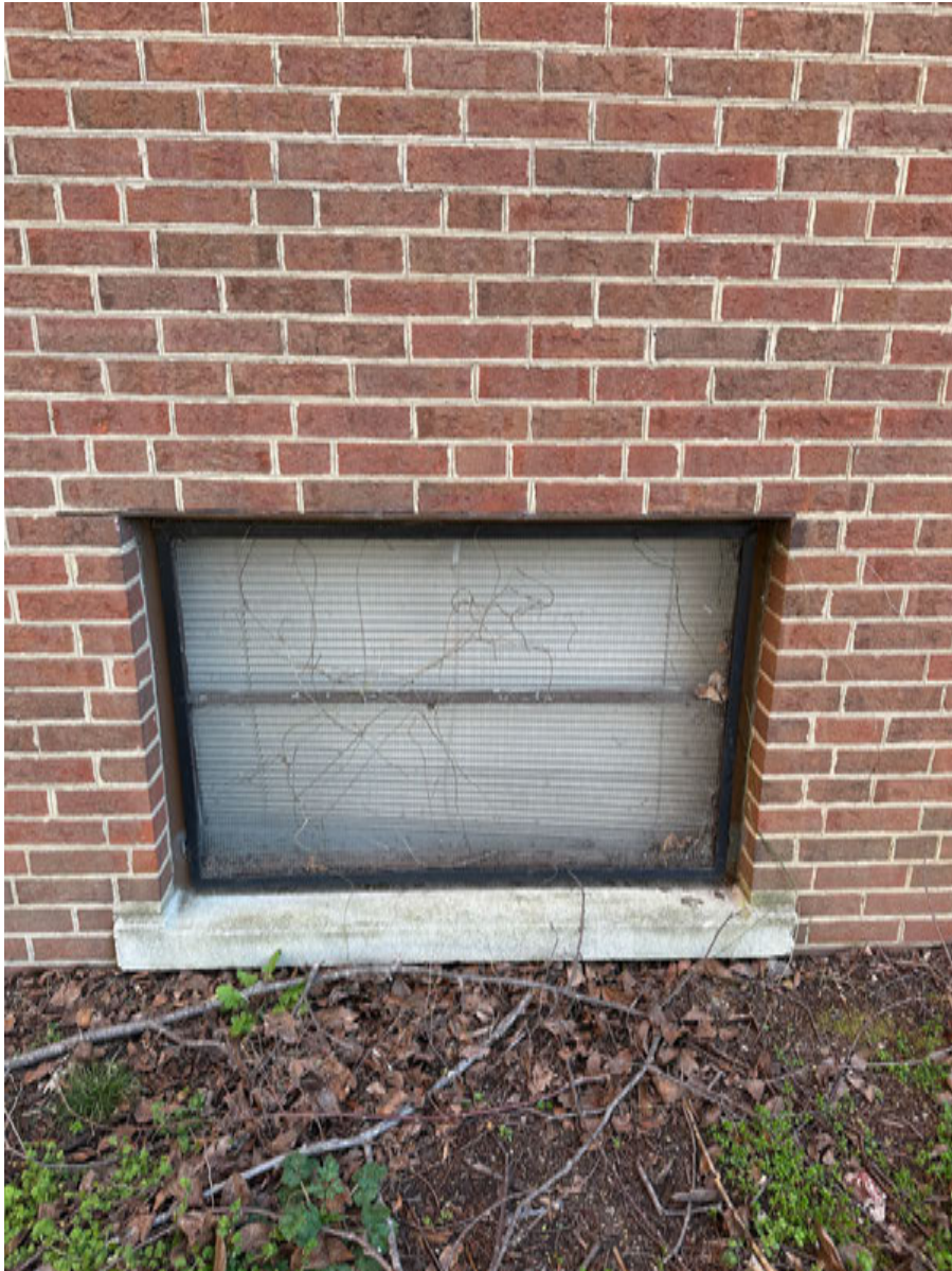
PHOTO: 2 W1 — West Elevation
