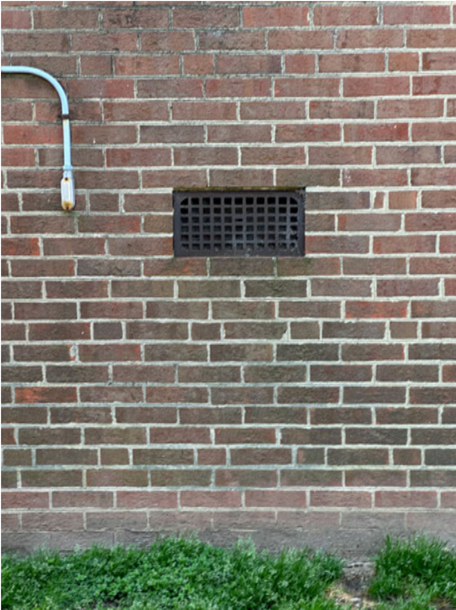
PHOTO: 9 E1 — East Elevation
