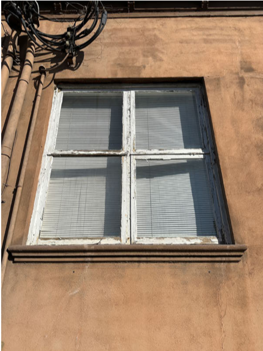
PHOTO: 5 S11 — South Elevation
