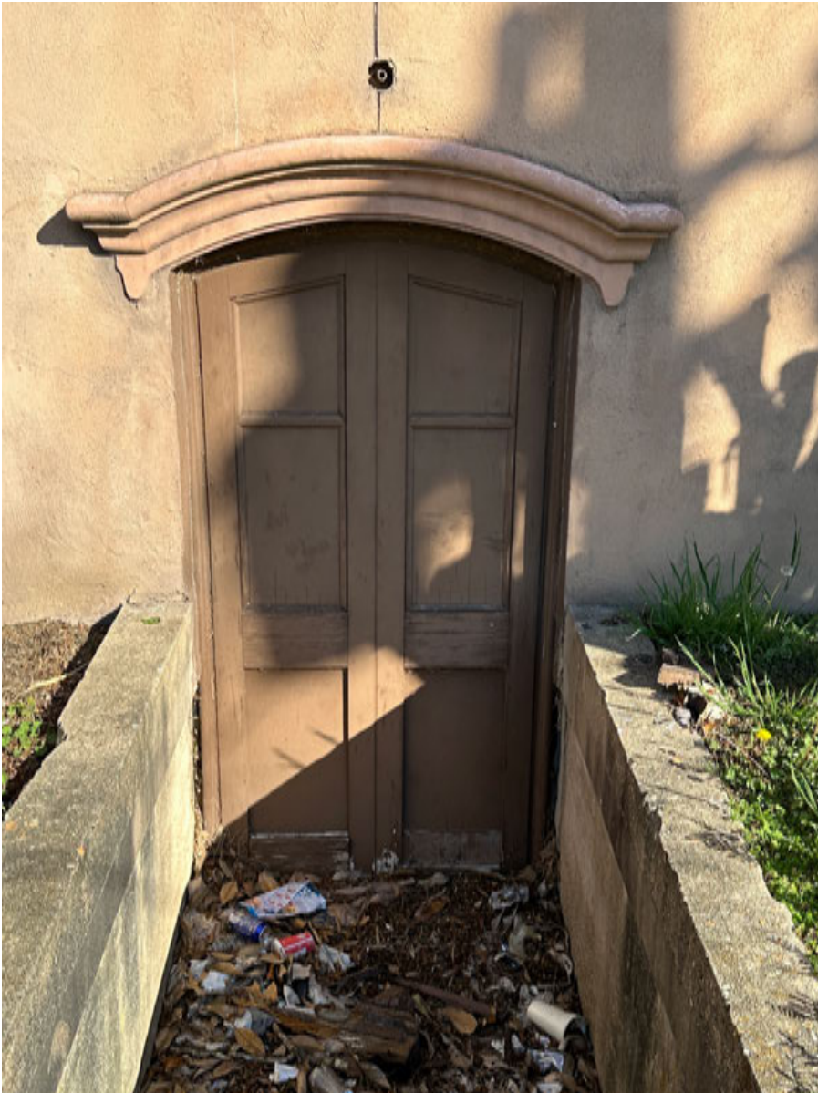
PHOTO: 5 S4 — South Elevation
