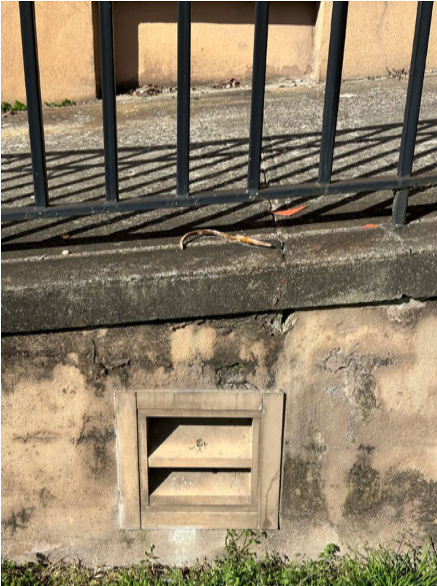
PHOTO: 7 E5 — East Elevation
