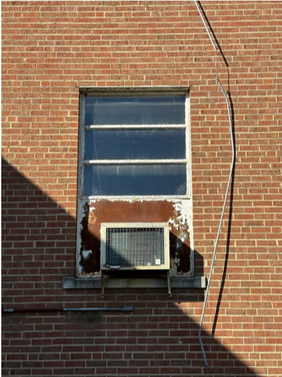
PHOTO: 9 E4 — East Elevation
