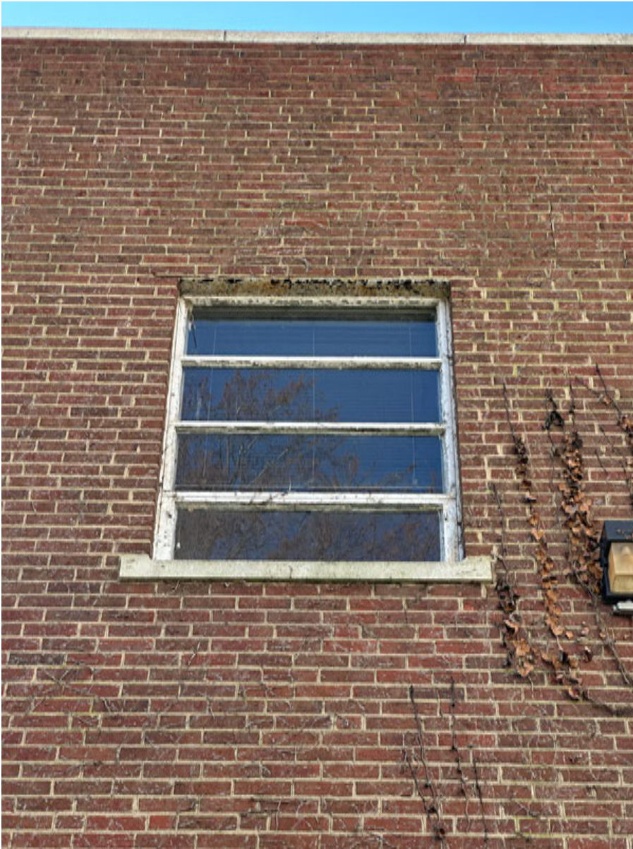
PHOTO: 10 N4 — North Elevation
