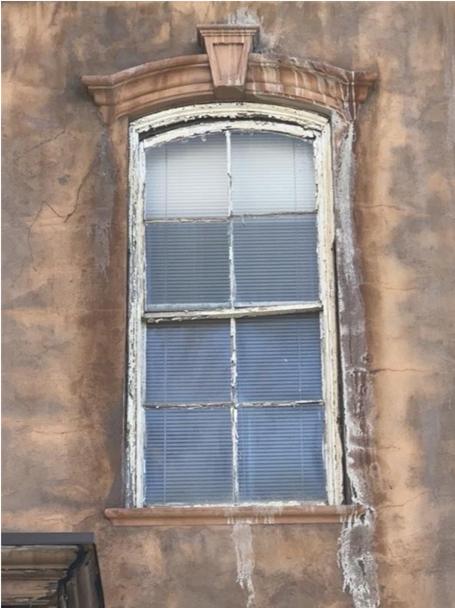
PHOTO: 1 W13 — West Elevation
