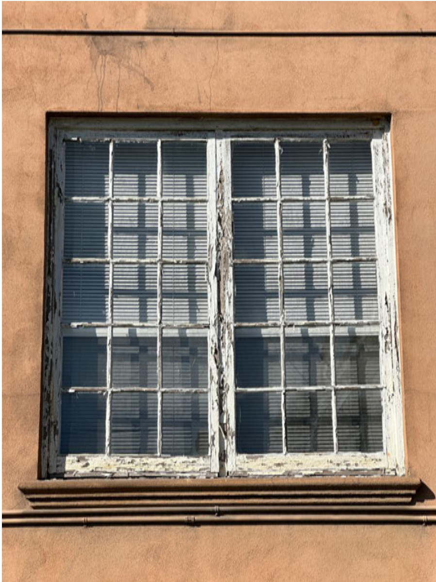
PHOTO: 7 E4 — East Elevation
