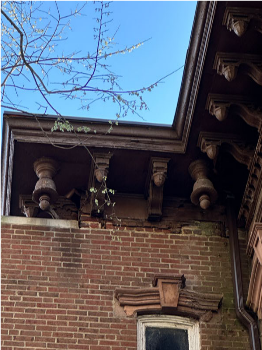
PHOTO: 2 W7 — West Elevation
