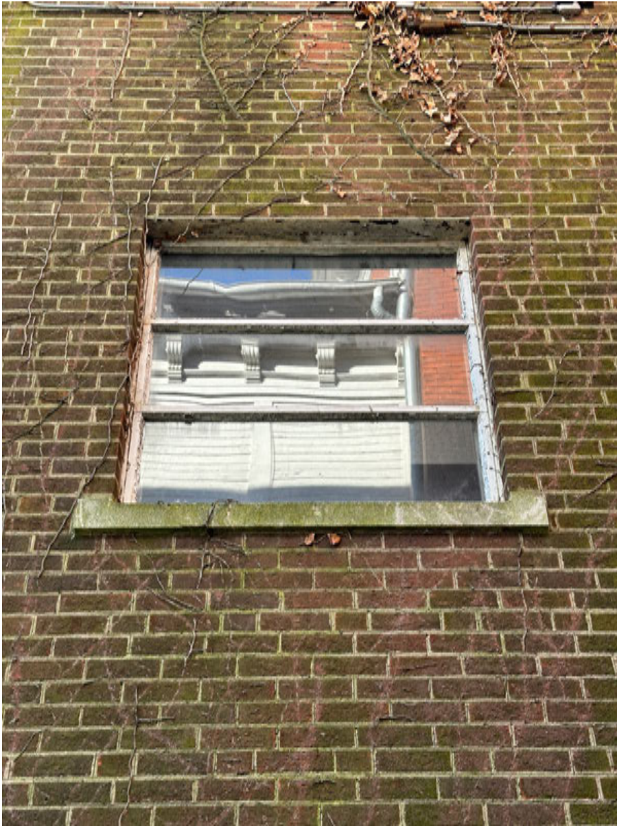
PHOTO: 11 N2 — North Elevation
