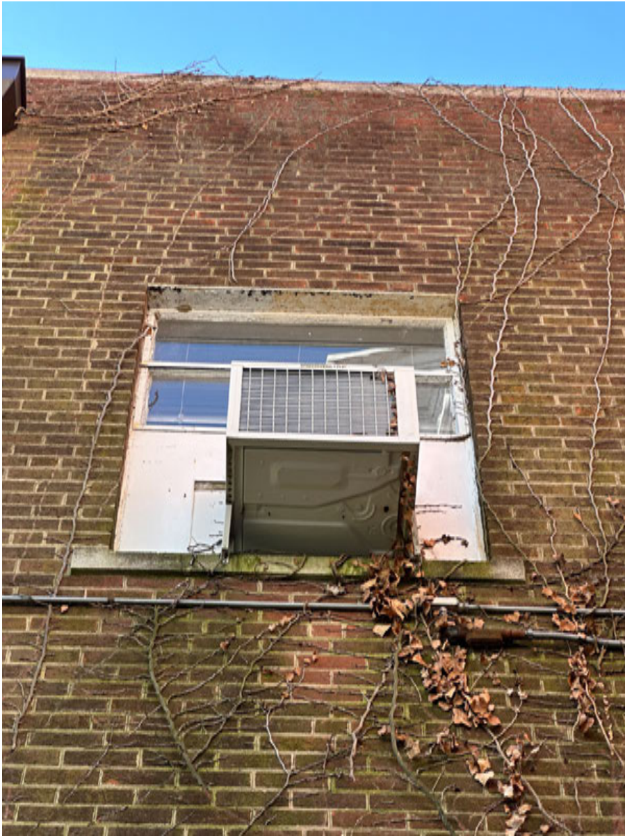
PHOTO: 11 N3 — North Elevation
