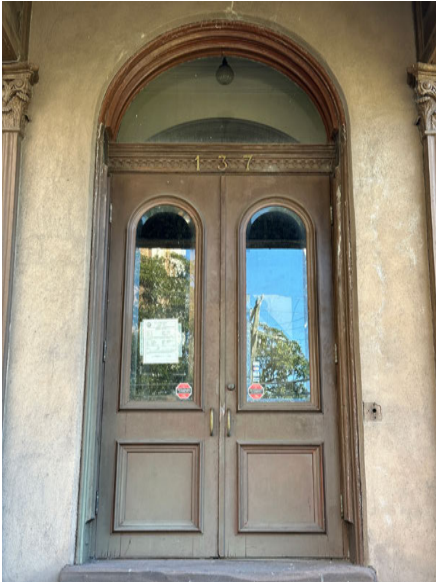
PHOTO: 1 W7 — West Elevation
