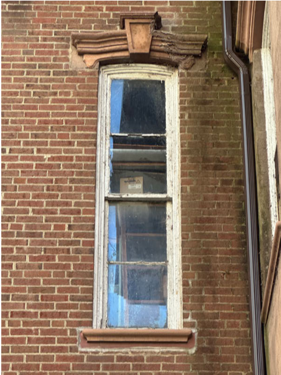
PHOTO: 2 W6 — West Elevation
