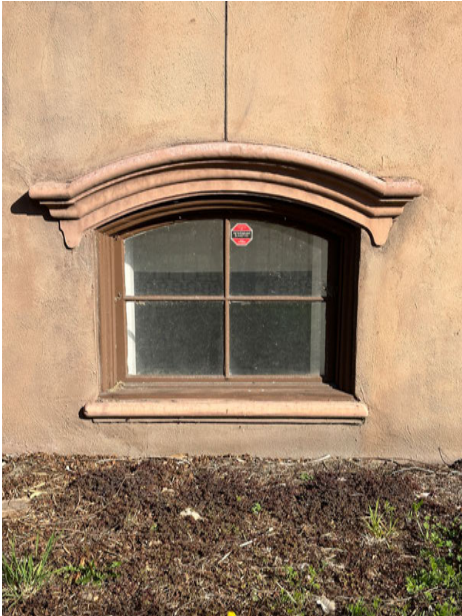
PHOTO: 5 S1 — South Elevation
