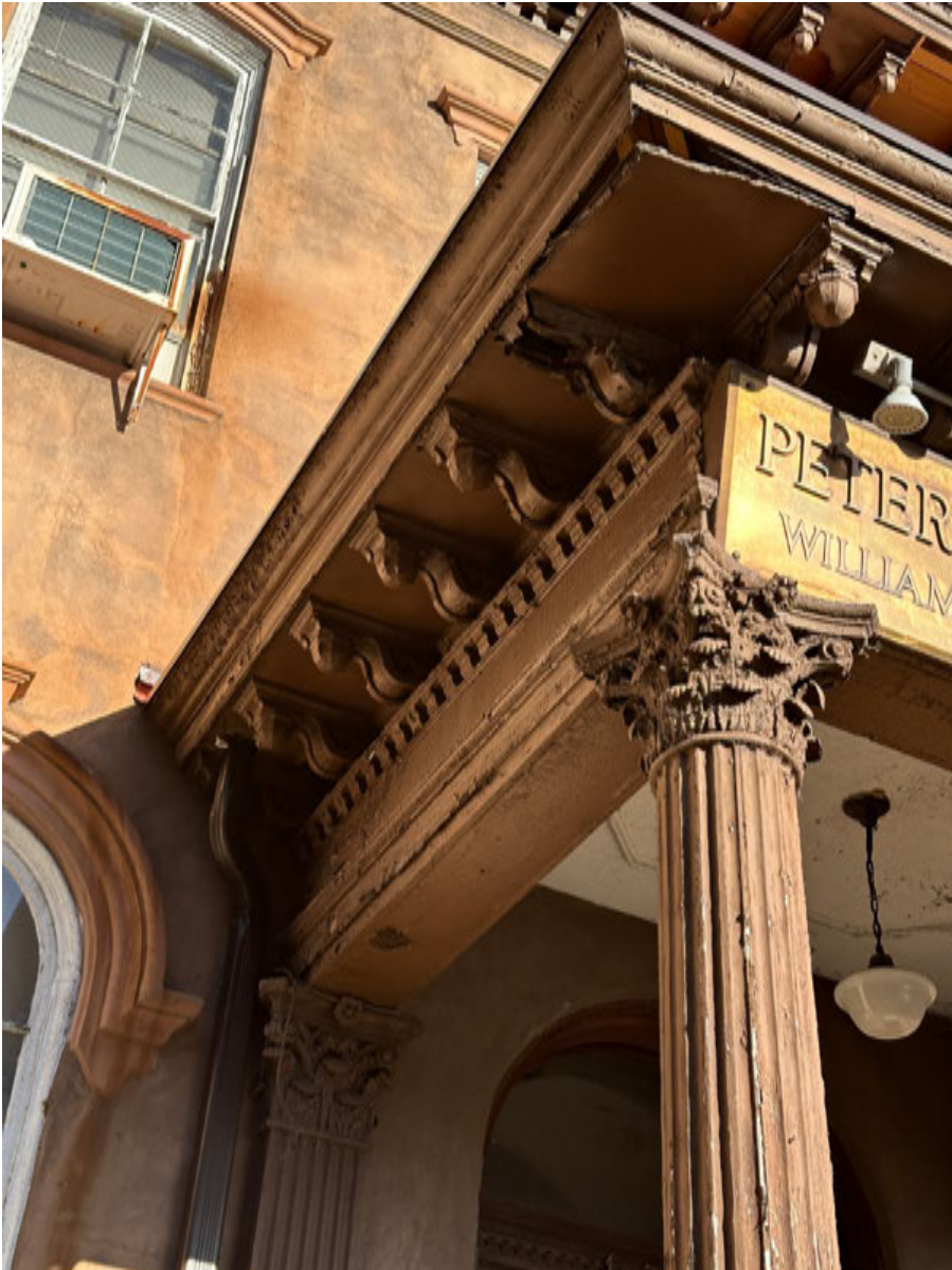
PHOTO: 1 W10 — West Elevation
