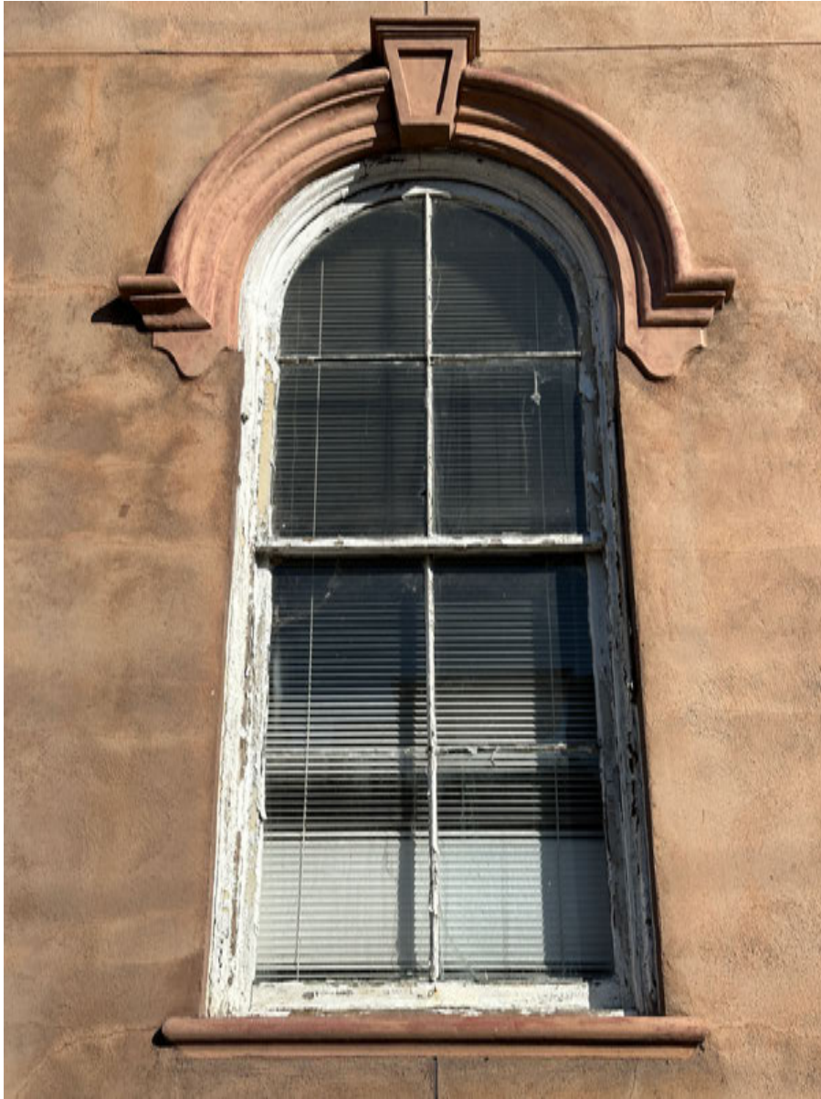
PHOTO: 5 S2 — South Elevation
