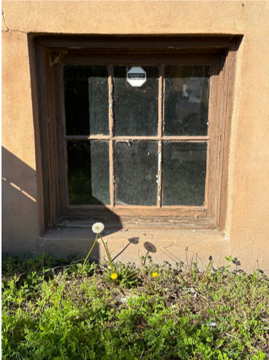
PHOTO: 5 S10 — South Elevation
