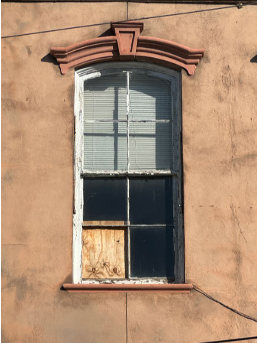
PHOTO: 5 S3 — South Elevation
