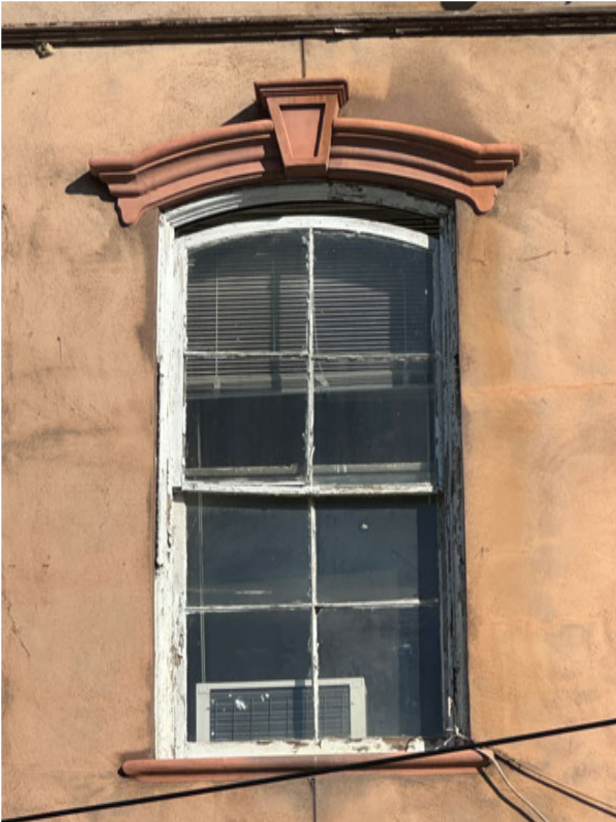
PHOTO: 5 S6 — South Elevation
