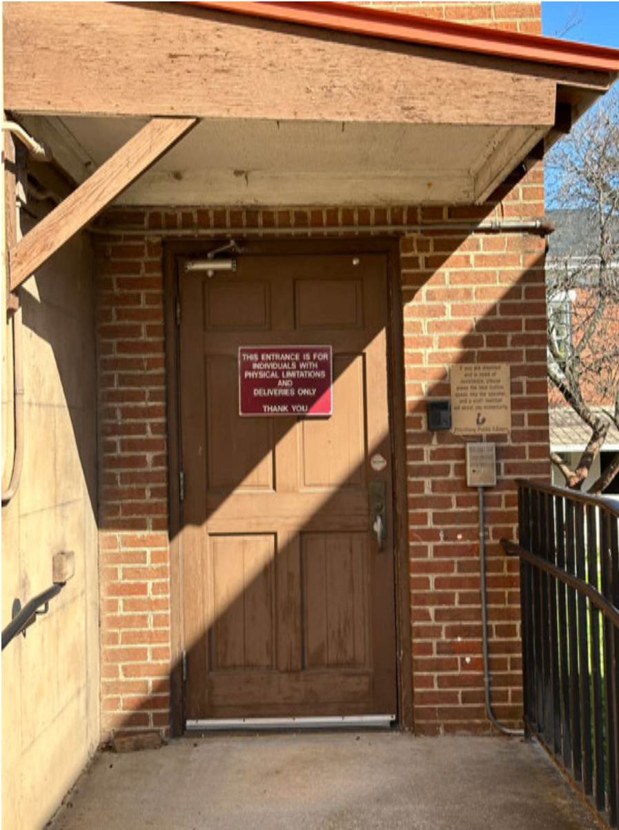
PHOTO: 6 S1 — South Elevation
