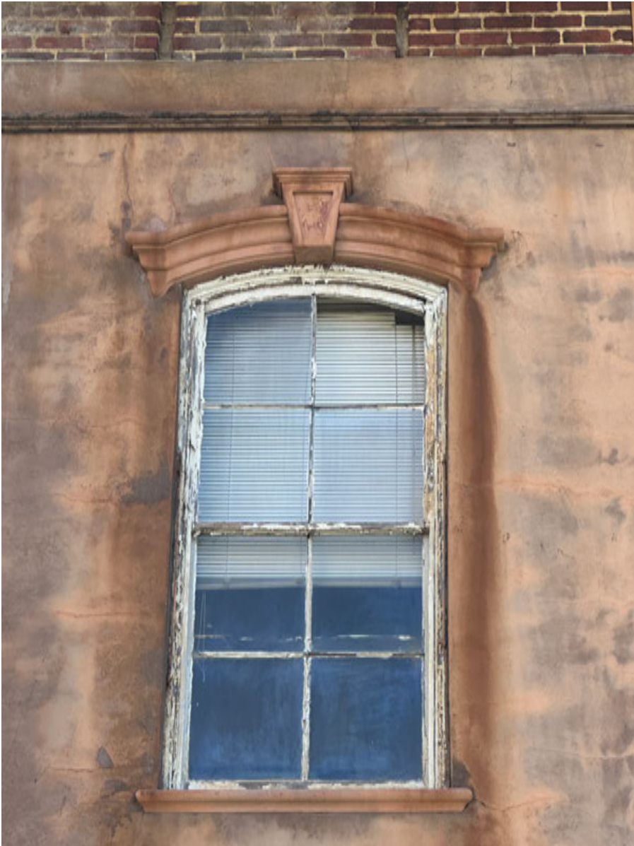
PHOTO: 1 W14 — West Elevation
