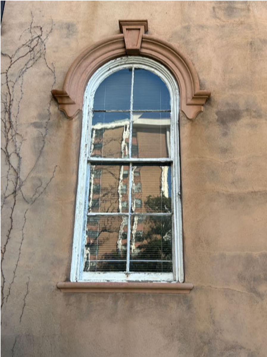
PHOTO: 1 W2 — West Elevation
