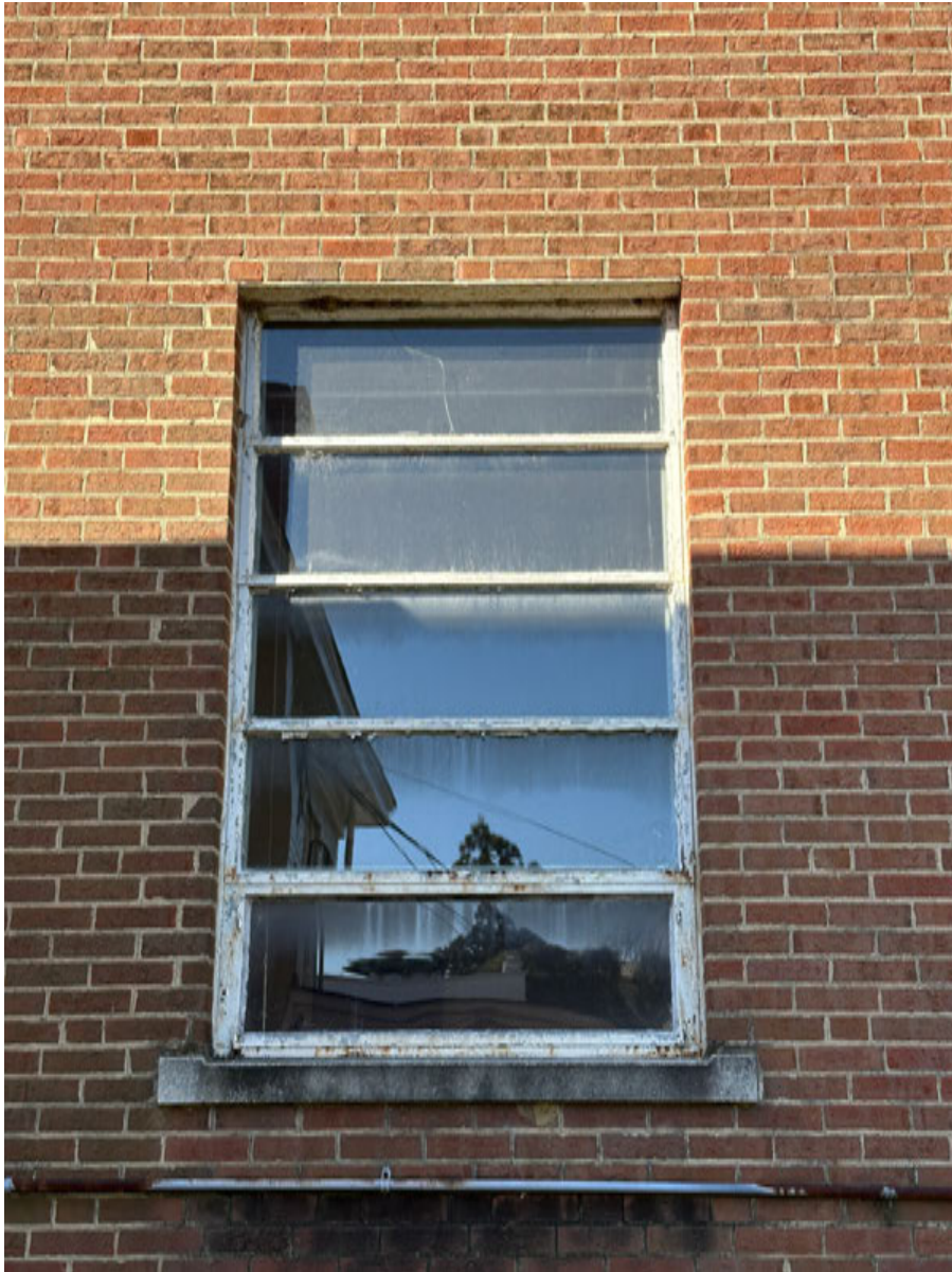
PHOTO: 9 E2 — East Elevation
