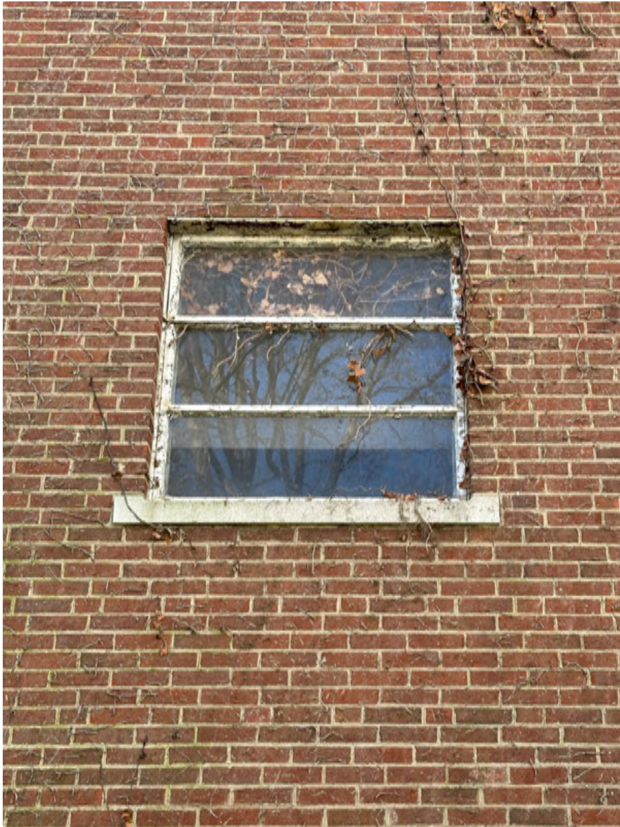
PHOTO: 10 N1 — North Elevation
