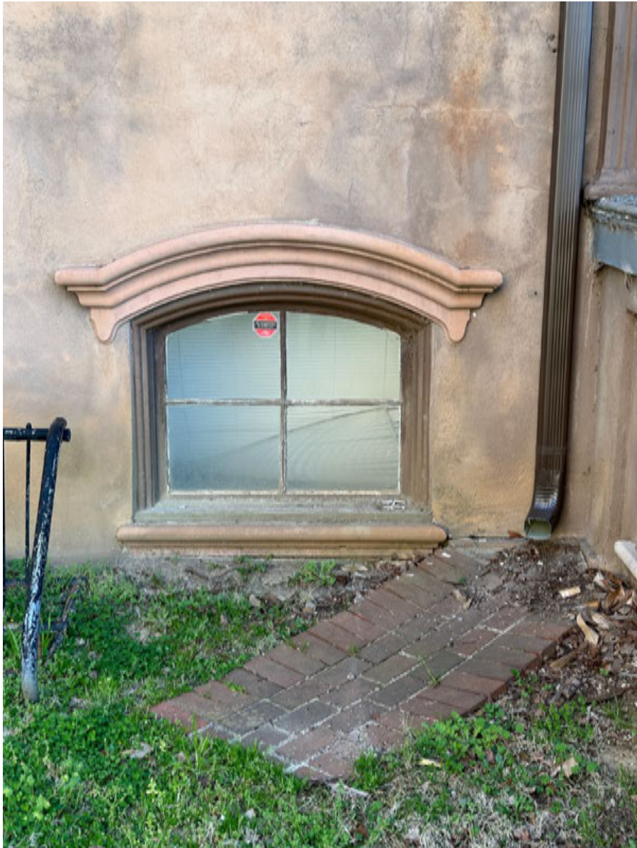
PHOTO: 1 W4 — West Elevation
