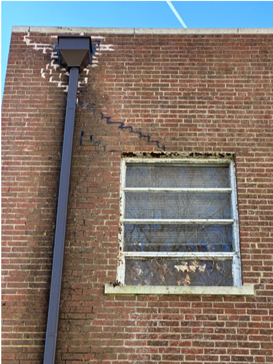
PHOTO: 10 N2 — North Elevation
