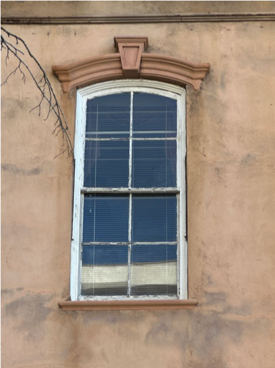
PHOTO: 1 W3 — West Elevation
