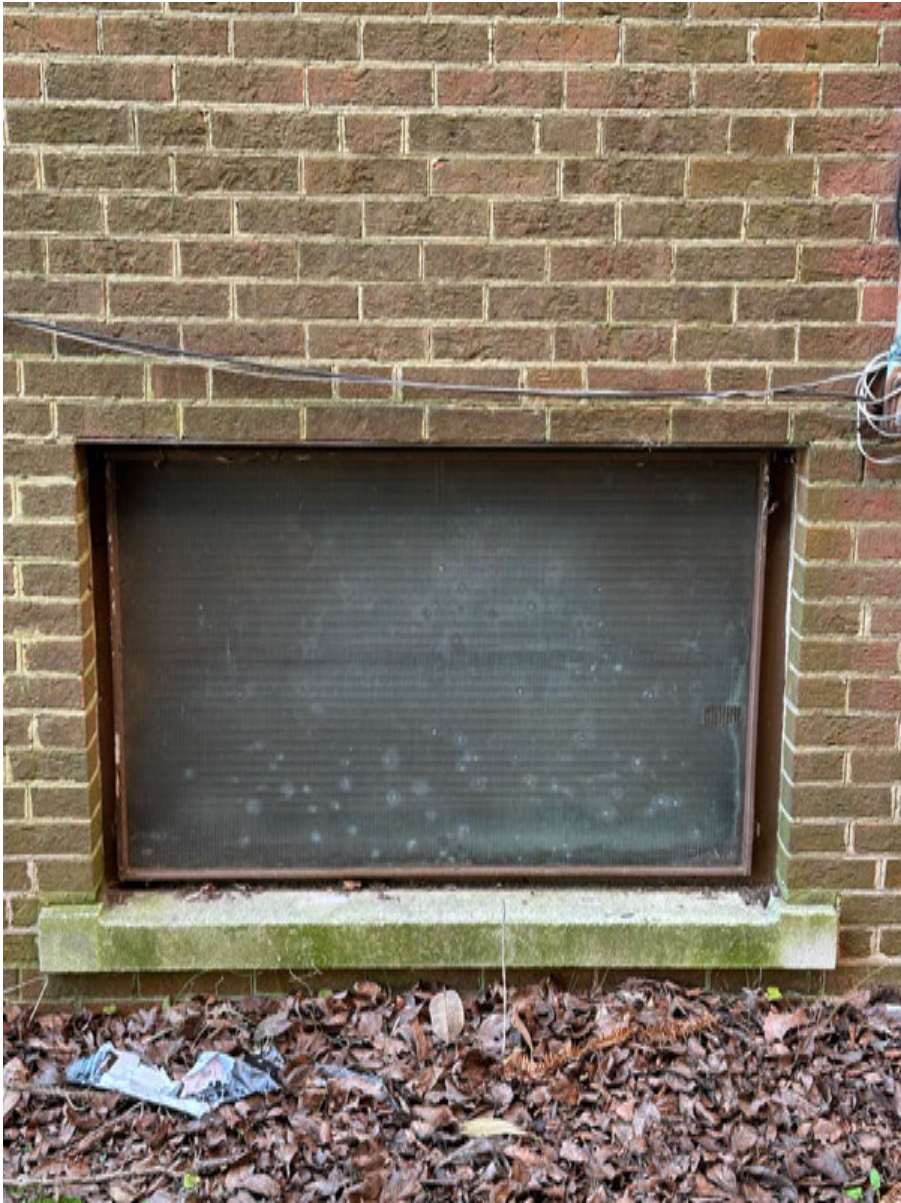
PHOTO: 11 N1 — North Elevation
