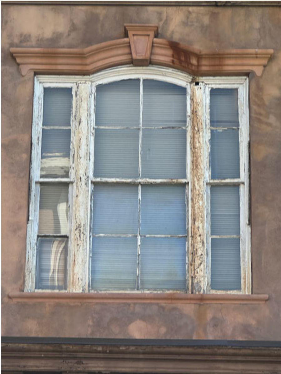
PHOTO: 1 W12 — West Elevation
