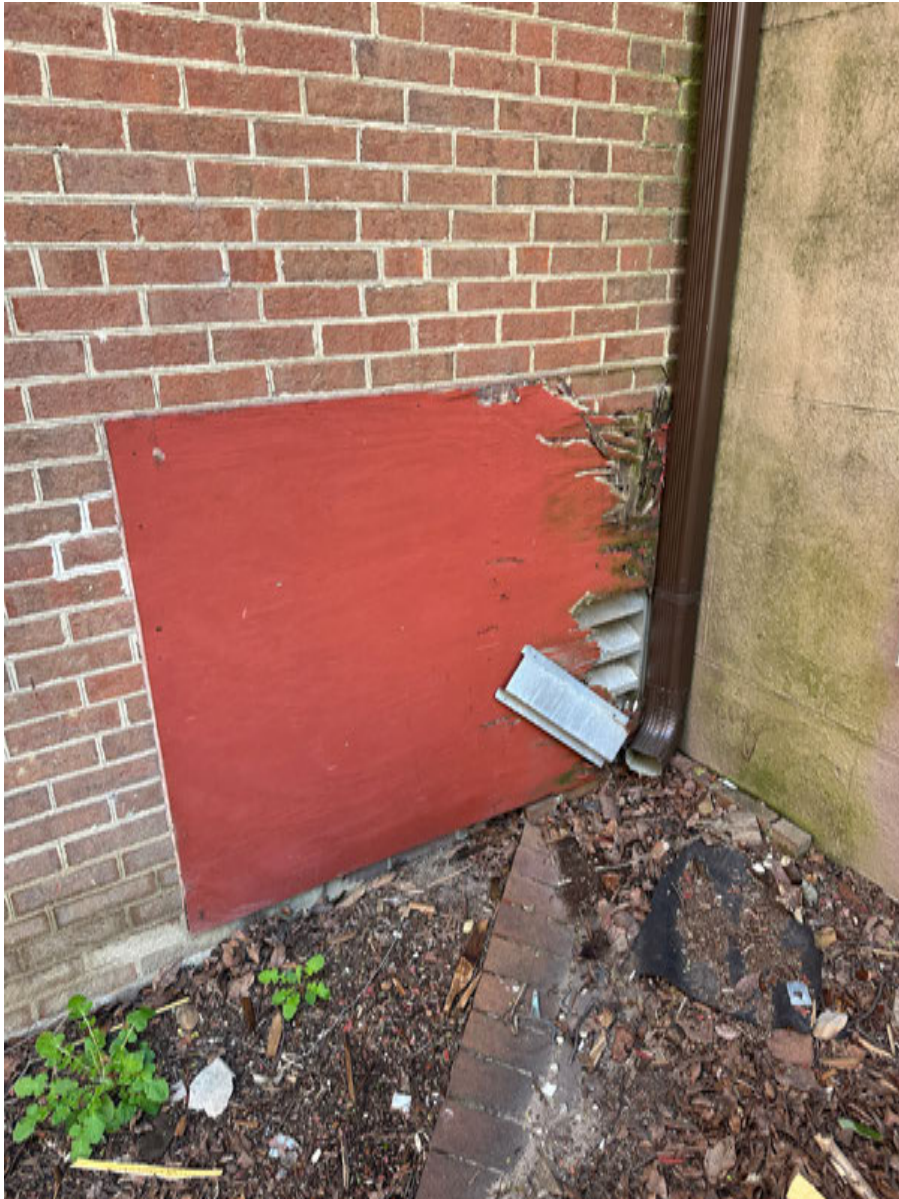
PHOTO: 2 W5 — West Elevation
