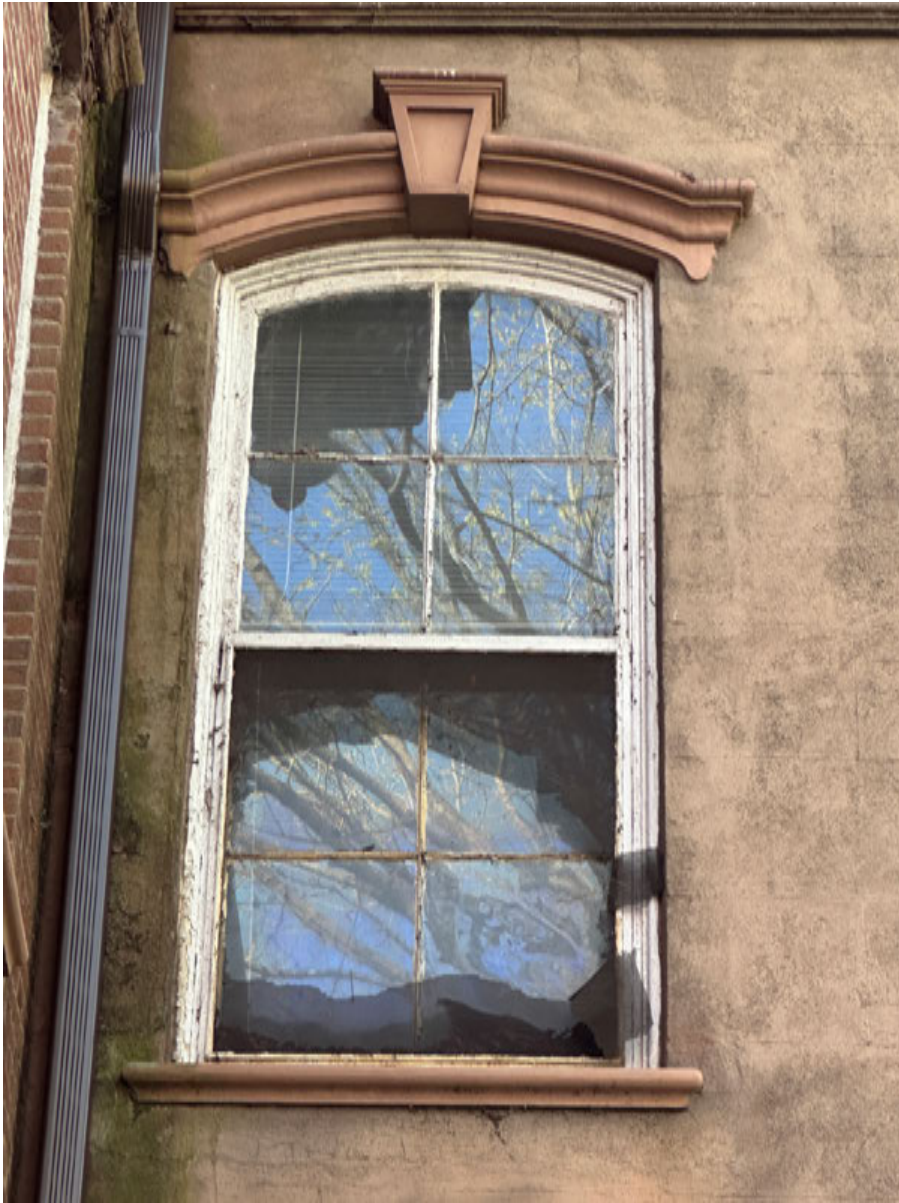
PHOTO: 12 N1 — North Elevation
