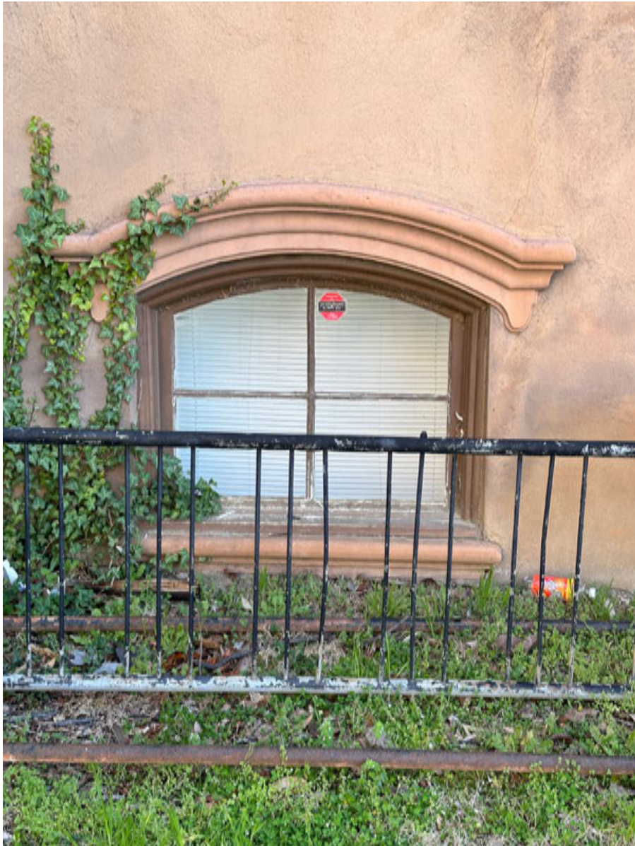
PHOTO: 1 W1 — West Elevation
