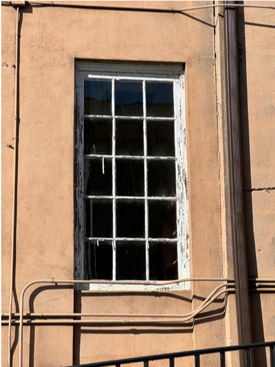
PHOTO: 7 E7 — East Elevation
