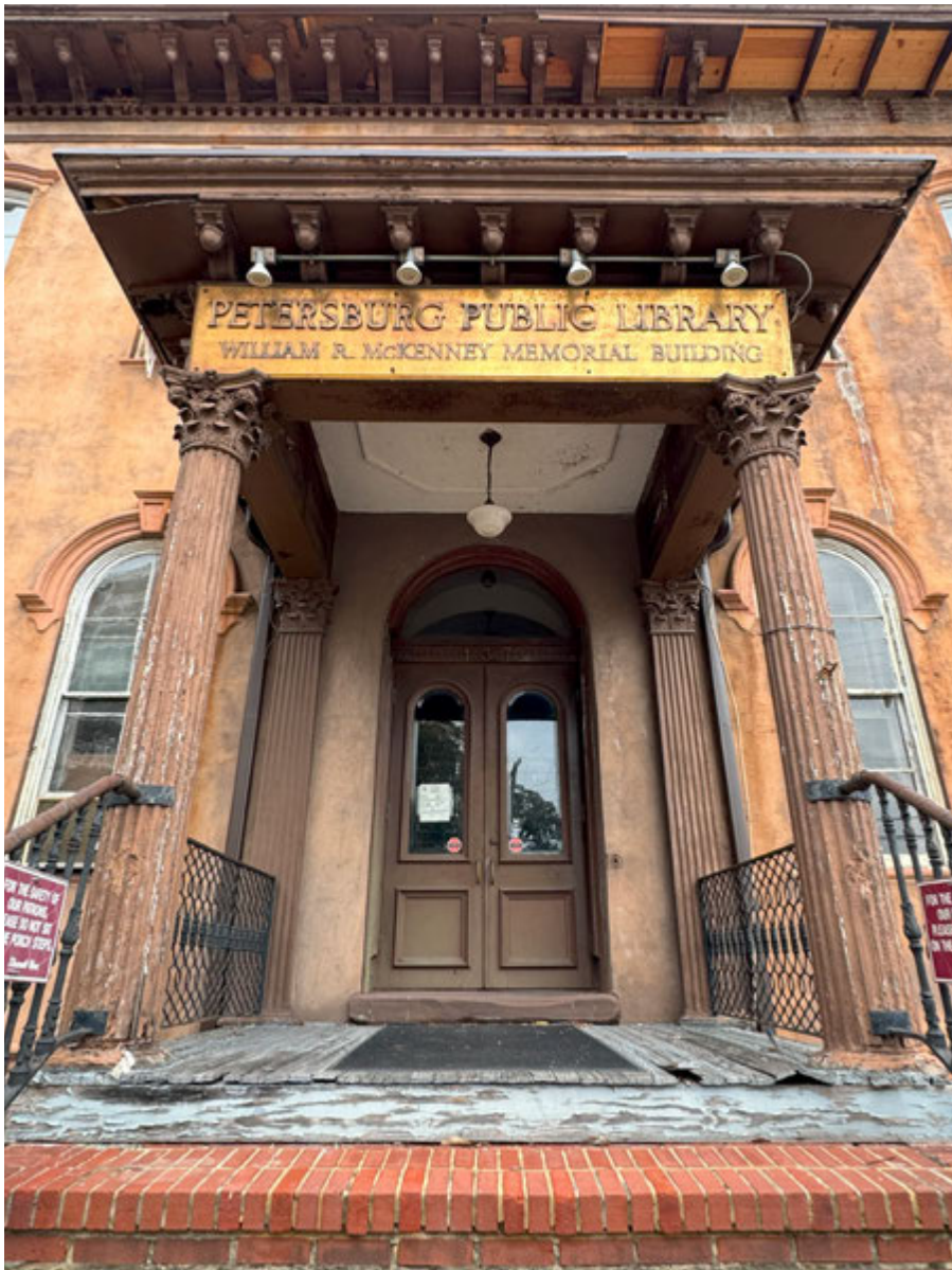
PHOTO: 1 W8 — West Elevation
