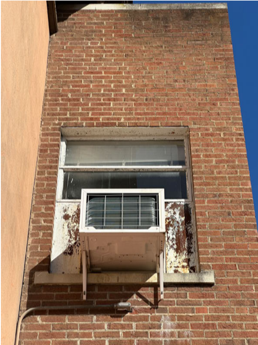
PHOTO: 6 S2 — South Elevation
