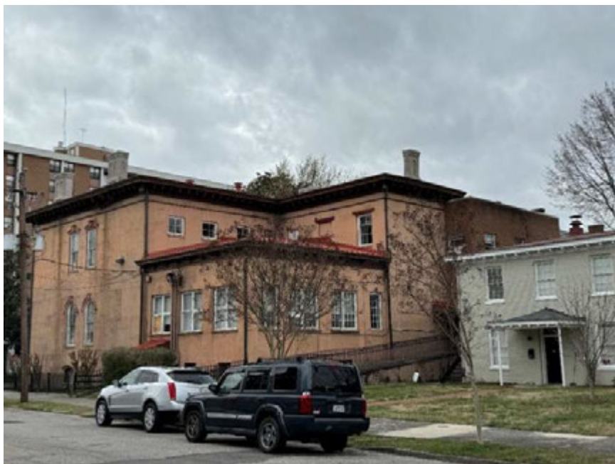
Photograph 2: Rear (East) Elevation
