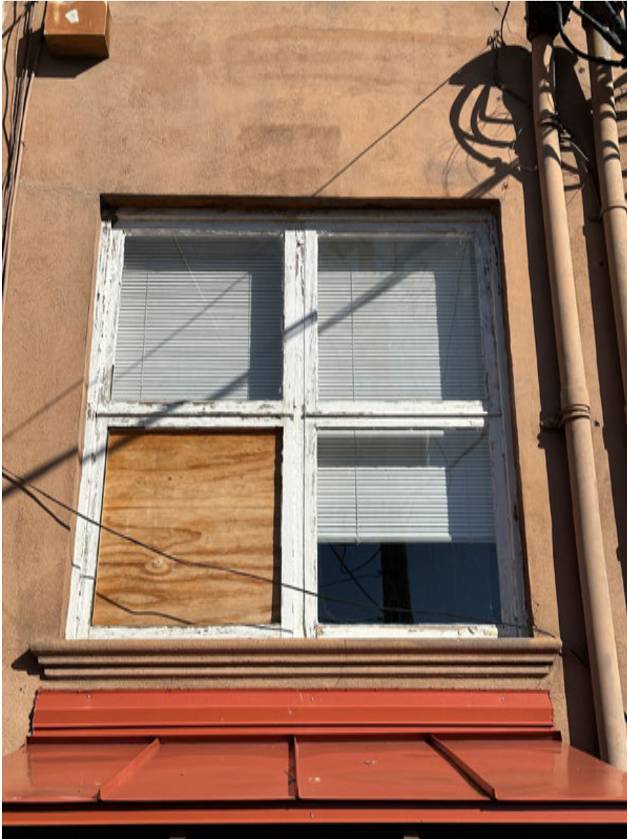
PHOTO: 5 S9 — South Elevation
