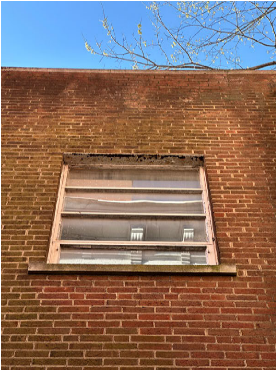
PHOTO: 11 N4 — North Elevation
